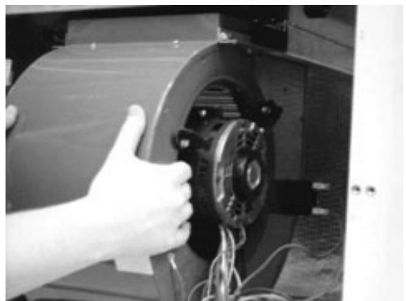
Removing the Supply Blower
