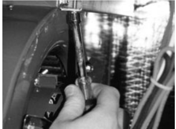
Removing the Supply Blower
